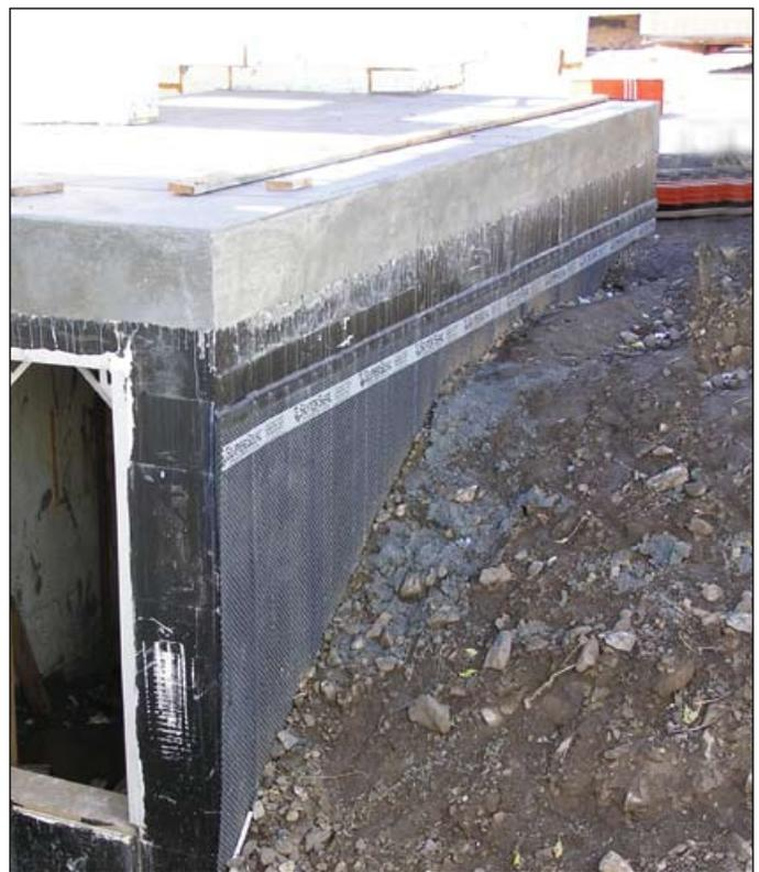
*Some dimple drain products utilize a fastening strip at the upper termination to prevent water from getting behind the membrane at grade.*
