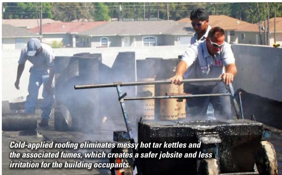
*Cold-applied roofing eliminates messy hot tar kettles and the associated fumes, which creates a safer jobsite and less irritation for the building occupants.*
