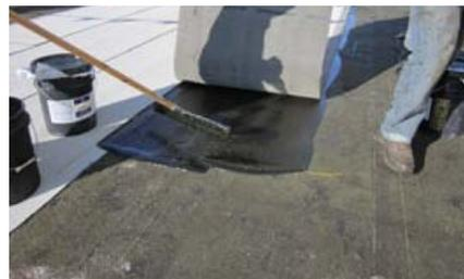
*An adaptation of “torch-down” roofing, cold modified bitumen roofs eliminate the torch and use adhesives to ensure the membrane and the substrate are sufficiently bonded.*
