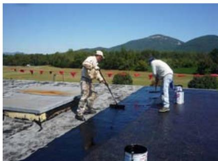
*Cold-process BUR uses solvent-based asphalt adhesives to adhere multiple layers of base sheet without heat. The membrane is then covered with aggregate.*
