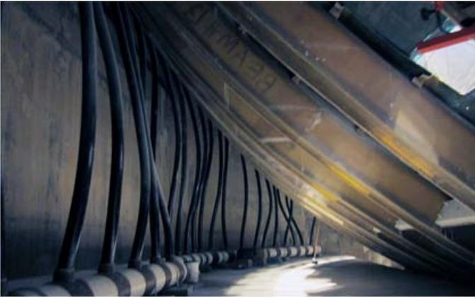
The large support ribs of the liner, seen here from the rear side, are also made of FRP. The original ribs were able to be reused for the new liner, even after 15 years in the water.
