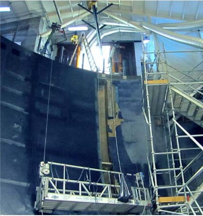
*Swing-stage scaffolding was used to install the new FRP panels on the existing rib structure.*
