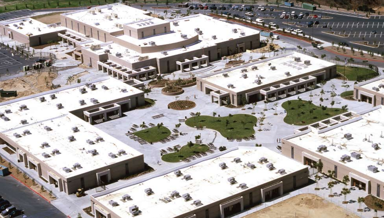
Photos Courtesy of Jay Thompson/Sarnafil
